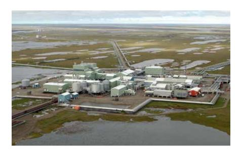
The Prudhoe Bay Field has more than 1,300 active oil-producing wells. Drilling is expected to continue for many years. Prudhoe Bay also is the site of one of the largest waterflood and enhanced oil recovery projects in the world, as well as a large gas processing plant that processes more than 7 BCFD of natural gas before reinjection into the reservoir.
