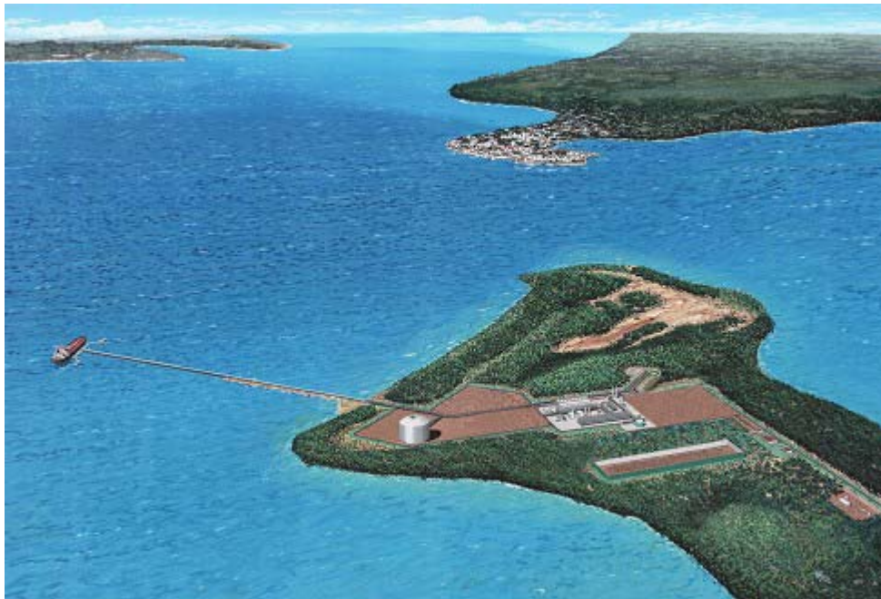
Figure 4 Darwin LNG Project, Wickham Point, Australia
