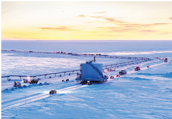
A tank is carefully transported along an ice road to the Willow field.
