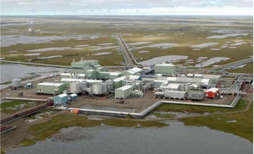
The Prudhoe Bay Field has more than 800 active oil-producing wells. Drilling is expected to continue for many years. Prudhoe Bay also is the site of one of the largest waterflood and enhanced oil recovery projects in the world, as well as a large gas processing plant that processes more than 7 billion cubic feet per day (BCFD) of natural gas before reinjection into the reservoir.
