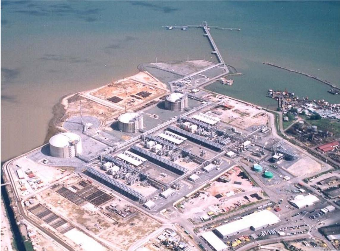
The fourth LNG train has been designed for a production capacity of nominally 5.2 MTPA. Included in the project is one additional 160,000 m<sup>3</sup> LNG tank and one additional jetty. Due to the perimeter constraints of the existing site, the newly constructed LNG Train needed to be optimized for the amount of land available at this location.
