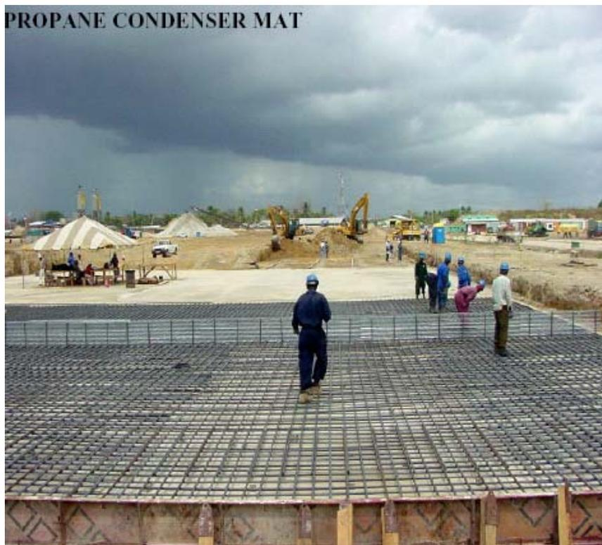
**Figure 7: Concrete Mats Process Area – June ‘03**
