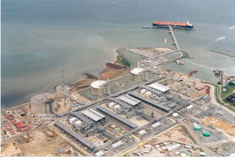
Figure 2: Construction continues on additional LNG capacity at the Atlantic LNG complex in Trinidad. Train 1 (on the right) has been operating successfully since July 1999. Train 2 was started up in August, 2002, 3 months ahead of schedule. Train 3 schedule has also been accelerated as well and it was started up in May 2003.
